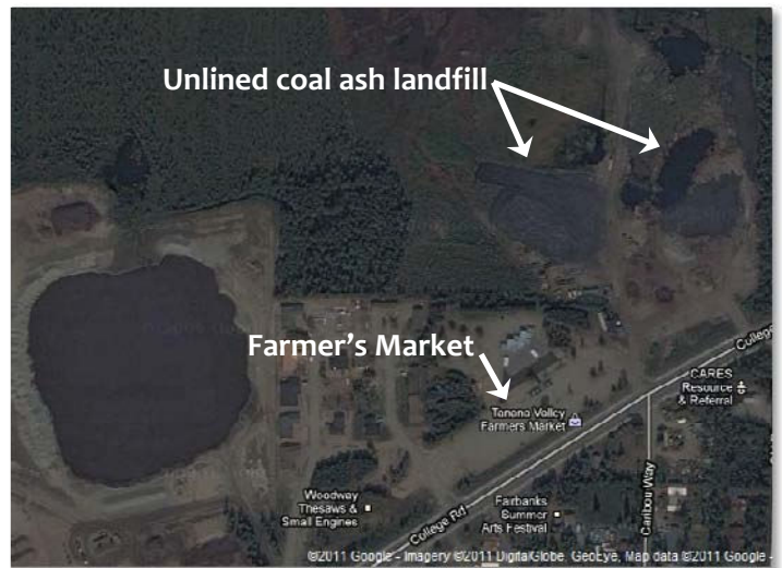
Location of Farmer's Market, showing proximity and size of neighboring coal ash landfill
