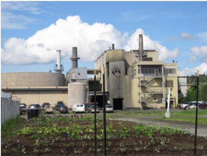
Garden planted in front of coal ash loading bay at UAF coal-fired power plant, June 2010
