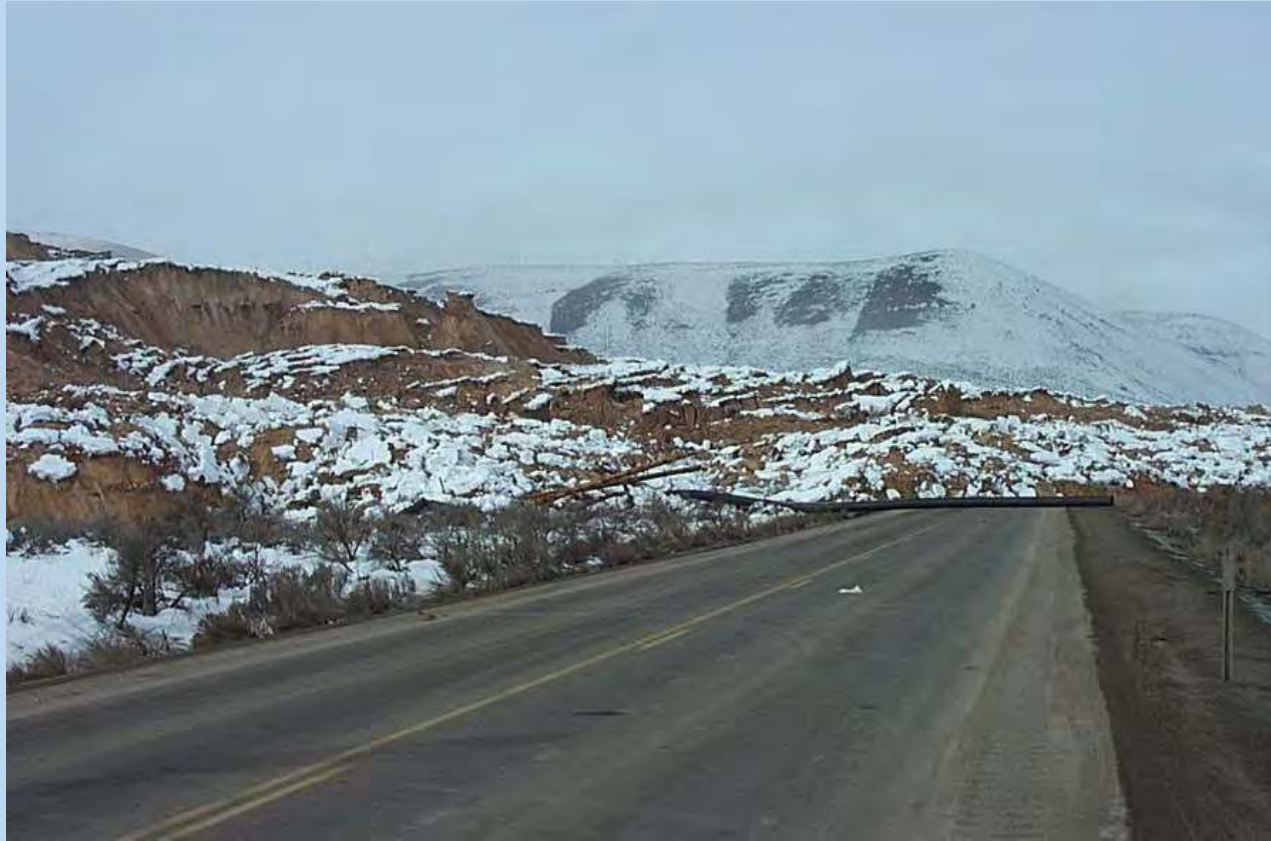
Gold Quarry Waste Rock Failure (Nevada)
